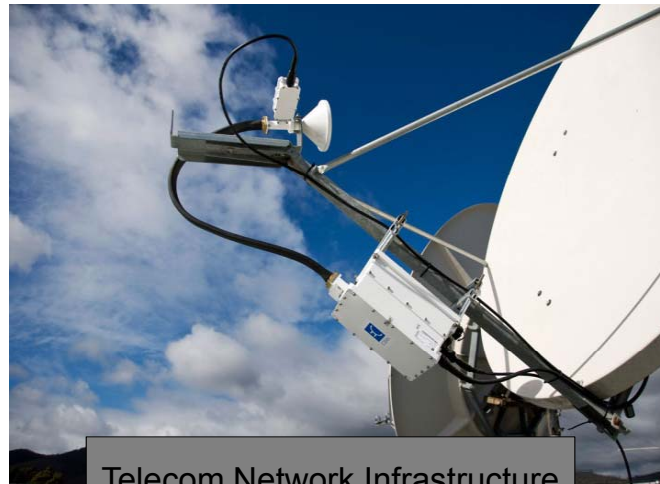
Telecom Network Infrastructure
