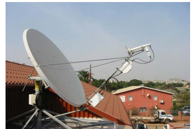
Antenna (With RF Subsystem mounted)
